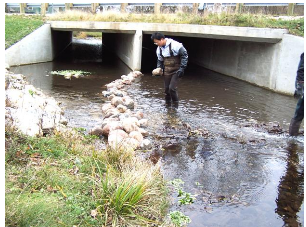
Stream improvements at the Highway LO bridge over Jericho Creek
